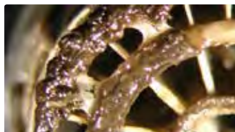
Water feeder with biofilm
